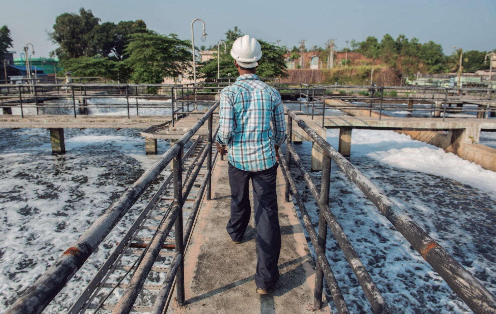
Kavoor Sewerage Treatment Plant in India. Photo/ADB_Creative Commons
